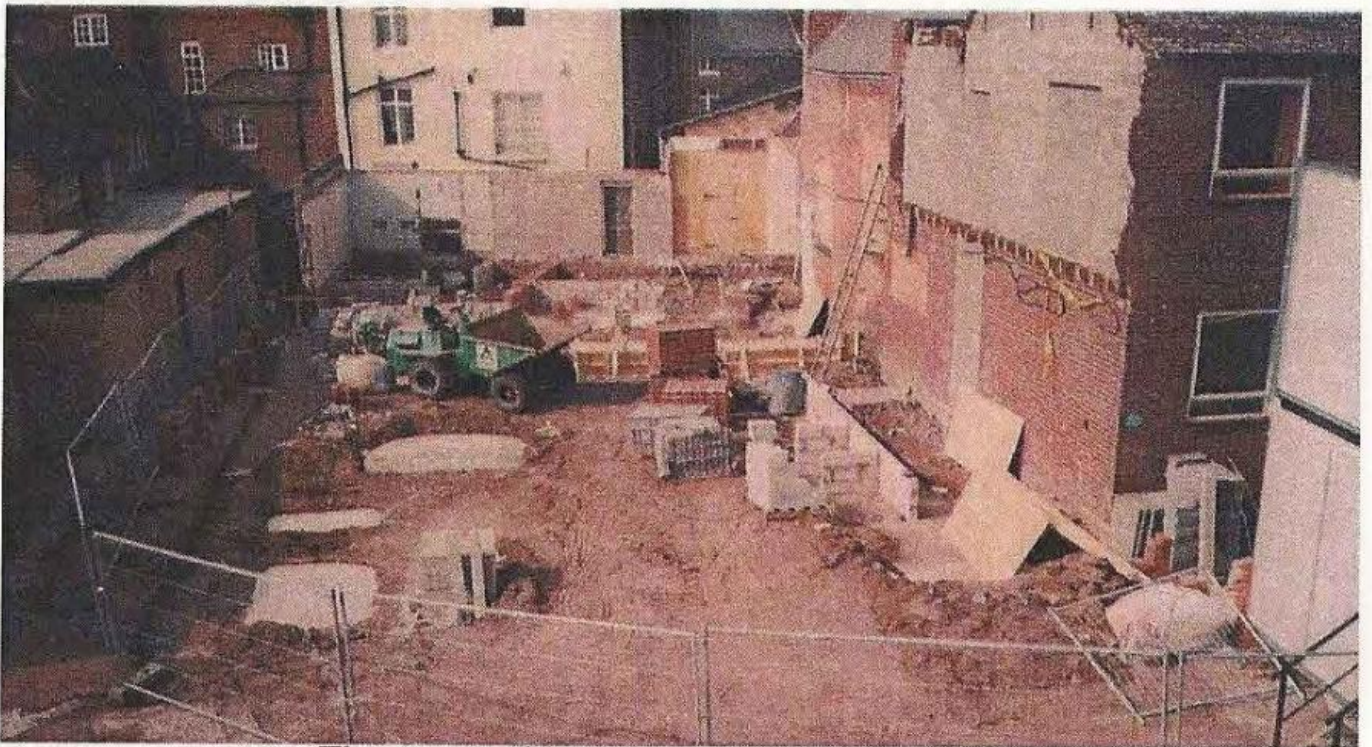
The start of building - September 1998
