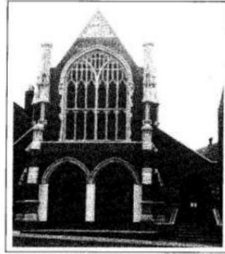
Exterior after 1982 alterations
